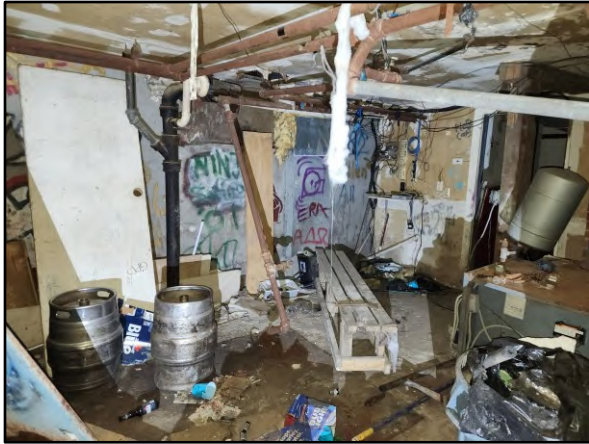
View of the basement utility room.
