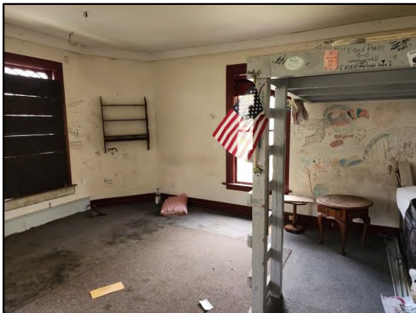
View of Bedroom 5 on the second floor.
