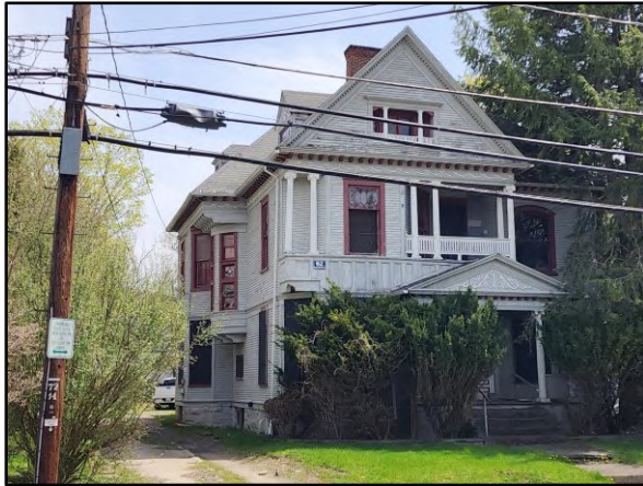
View of the exterior of the structure generally looking east.
