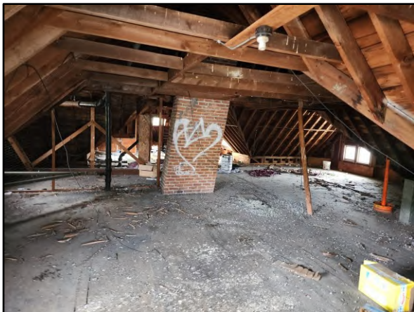
General view of the unfinished attic.
