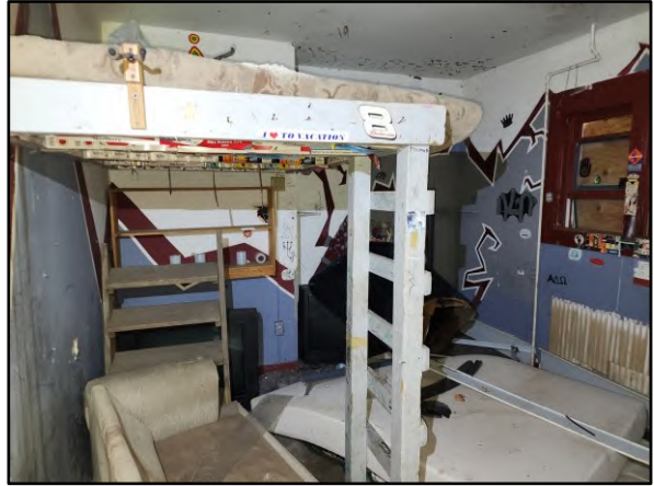
View of Bedroom 3 on the first floor.
