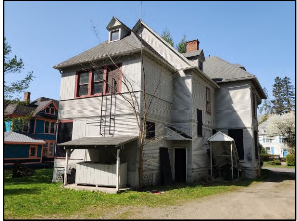
View of the exterior of the structure generally looking southwest.
