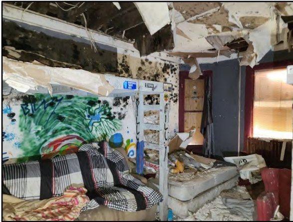
View of Bedroom 4 on the first floor.
