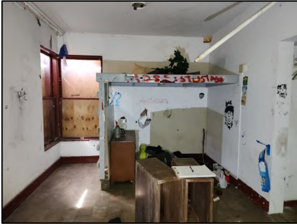
View of Bedroom 2 on the first floor.
