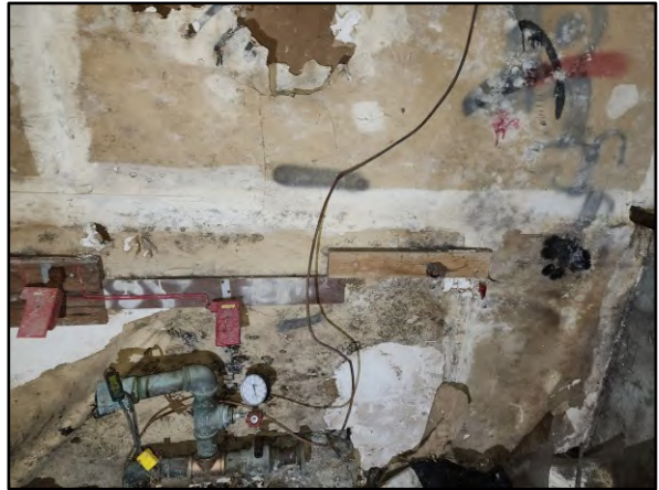
Mold on drywall wallboard in the basement.
