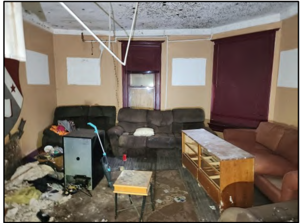
View of the first-floor living room.
