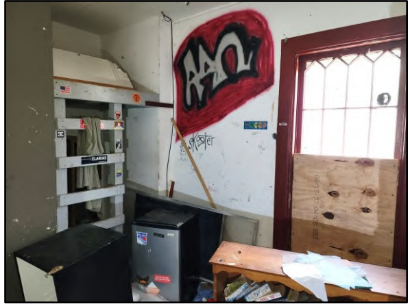
View of Bedroom 6 on the second floor.
