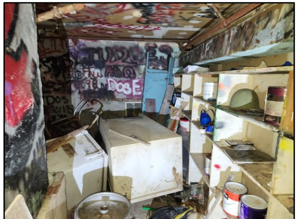
View of basement storage room 1.
