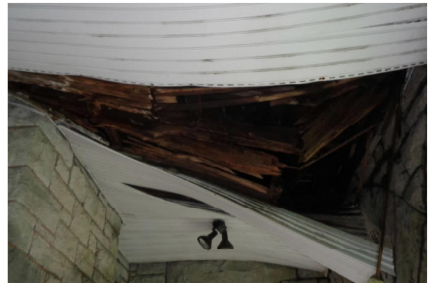
Fig. Ext-21. Porch Ceiling Damage.
