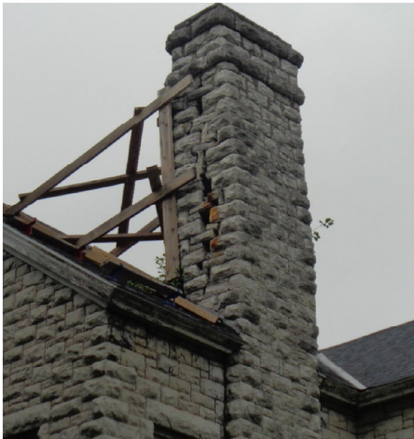
Fig. Ext-35. Main Chimney Deterioration.
