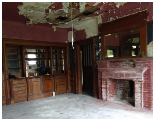
Fig. FF-18. Room 103 Ceiling/Wall Damage.
