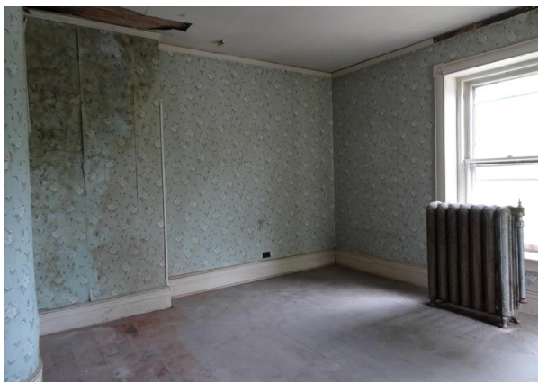
Fig. SF-24. Room 203 Water Infiltration Damage
