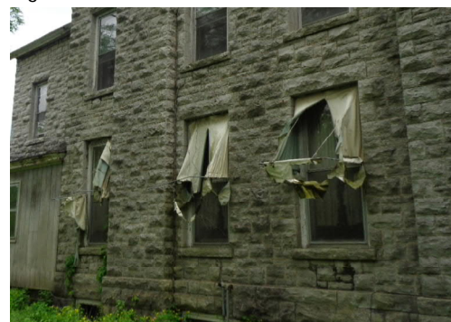
Fig. Ext-10. West Elevation Window Deterioration.
