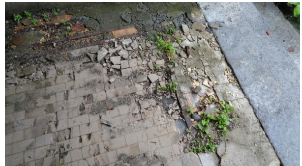
Fig. Ext-17. East Porch Tile Deterioration.
