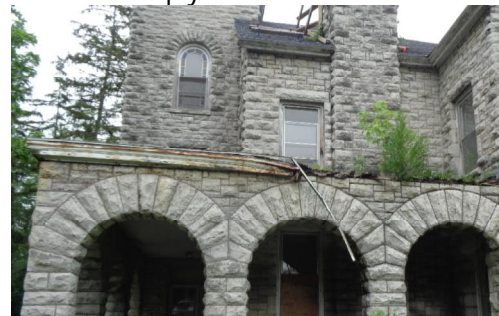
Fig. Ext-09. Porch Roof Deterioration.
