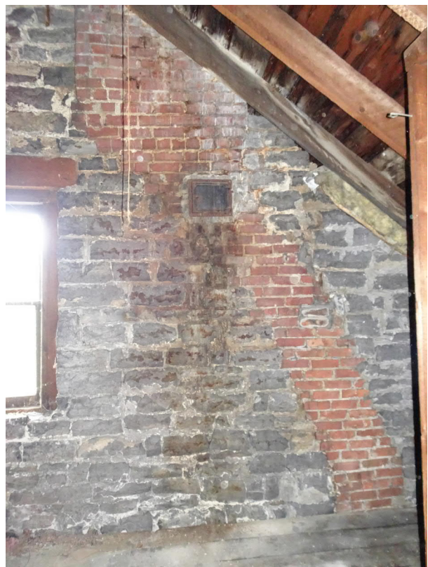
Fig. AT-30. West Attic Wall- Stone Damage.
