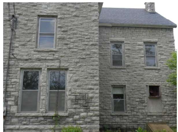
Fig. Ext-07. Stone Deterioration- East Facade.
